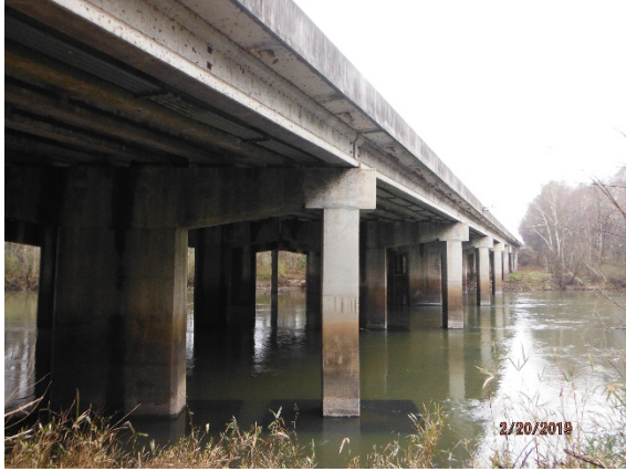
Photo 1. East Side View of bridge
