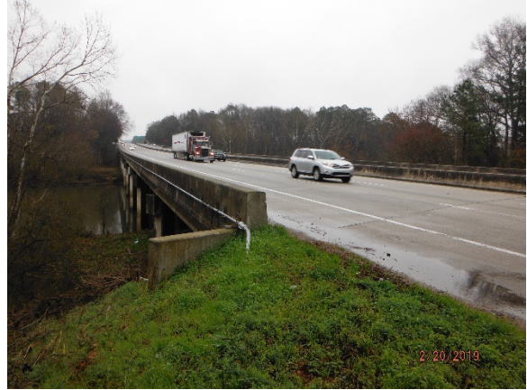
Photo 2. Top of Bridge Deck View
